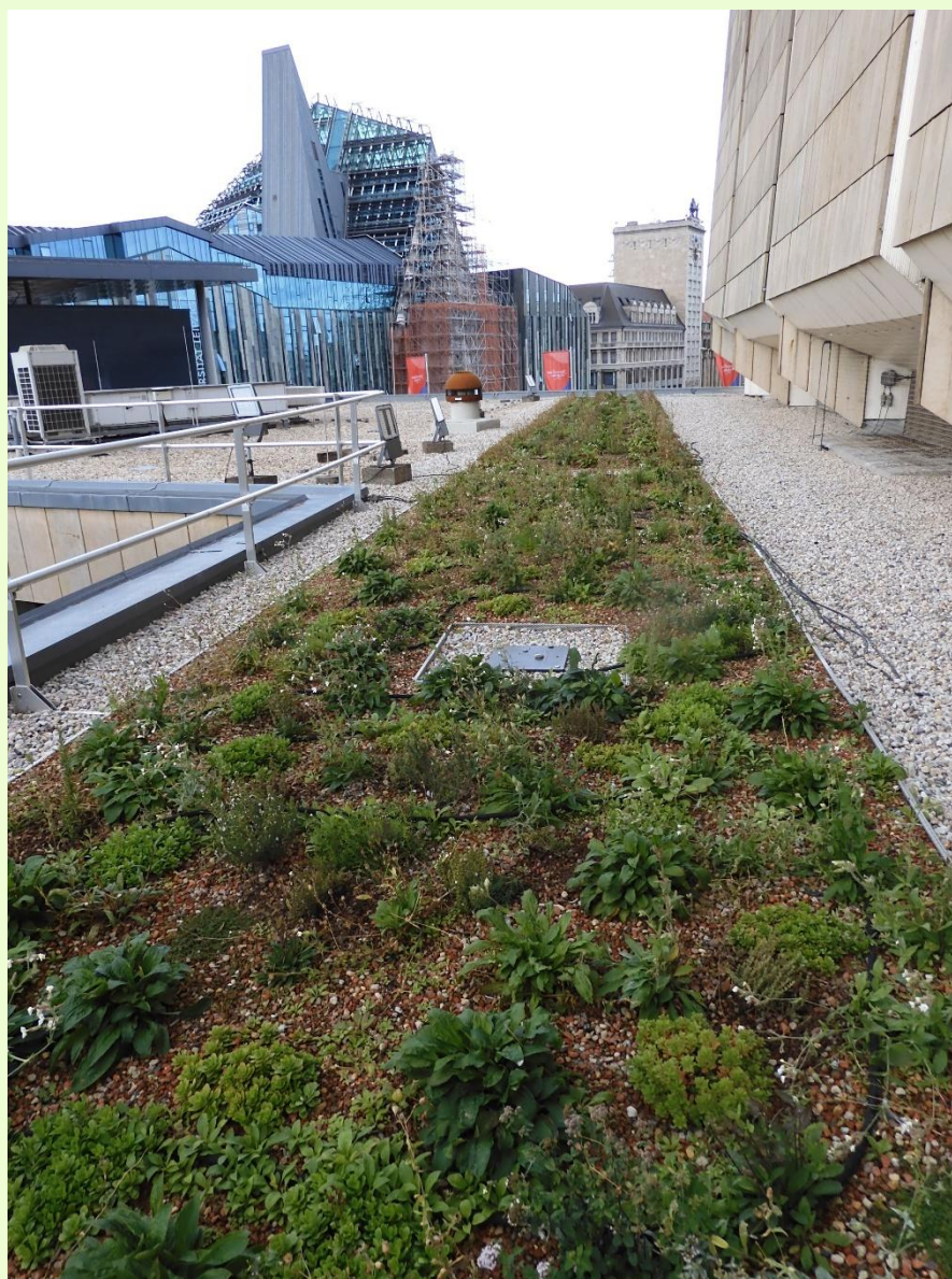
Figure 4: Green roof segment (extensively [front] and simply intensively planted) on the west side (photo taken on 24 September 2025).
